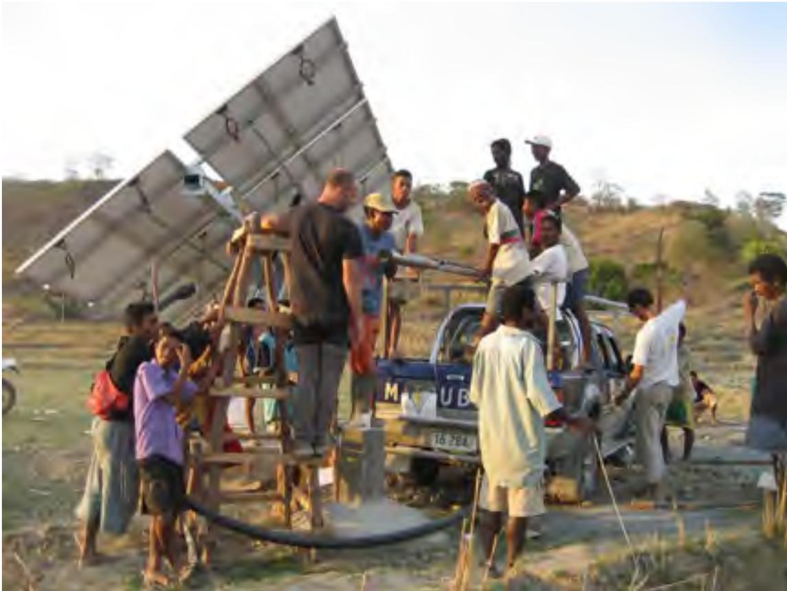
**Figure 18: Installation of submersible bore well pump and solar array in Cairui, East Timor.**
