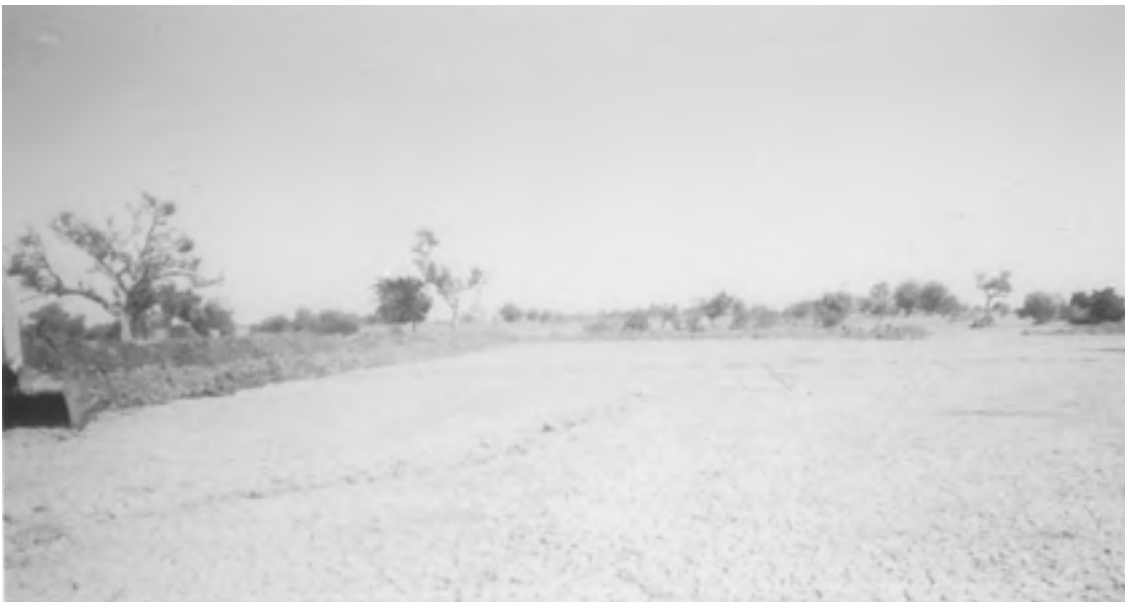
Figure 11 The Kamian Catchment excavation in progress (100m by 80m by 1.5m)
