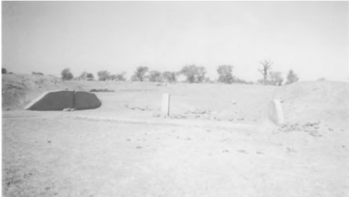
Figure 10 Village of Sagabugu Catchment's reinforced water entrance ramp
