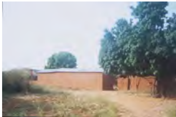
Figure 7 Types of roofs in Mali
