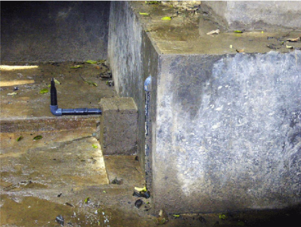
**Figure 11. Reservoir with Collection, Overflow, and Drainage Pipe.**
