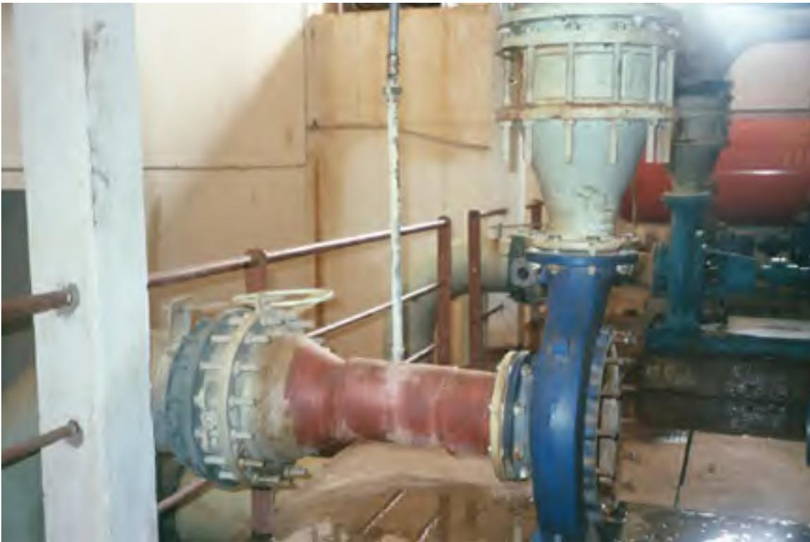
**Figure 3-9. Main pumps to the Kayes' Distribution System**
