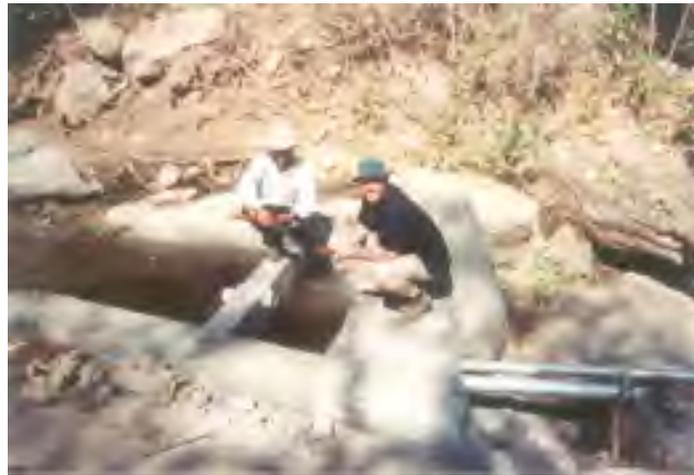
**Figure 3-3: Example of concrete surface-water source with settling chamber for community of 150 houses, feeding a tank of 10,000 gallons, with capacity of tubing to carry 50 gallons per minute. Approximate flow rate of source as shown = 75 gallons per minute.**
