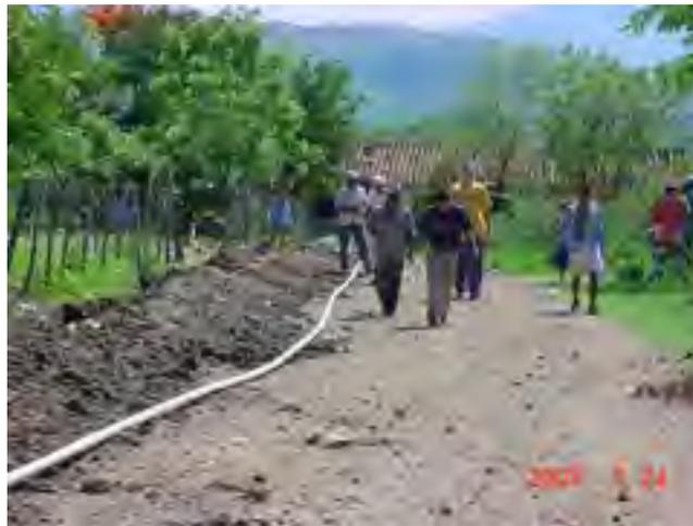
**Figure 3-6: 2” PVC tubing ready to be placed in 3’ deep trench for distribution line in a community of 50 houses.**
