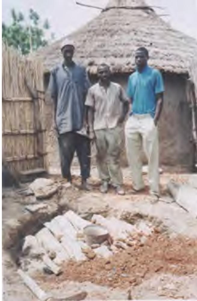
**Figure 4.12: Wood Slab of Traditional Latrine Floor**
