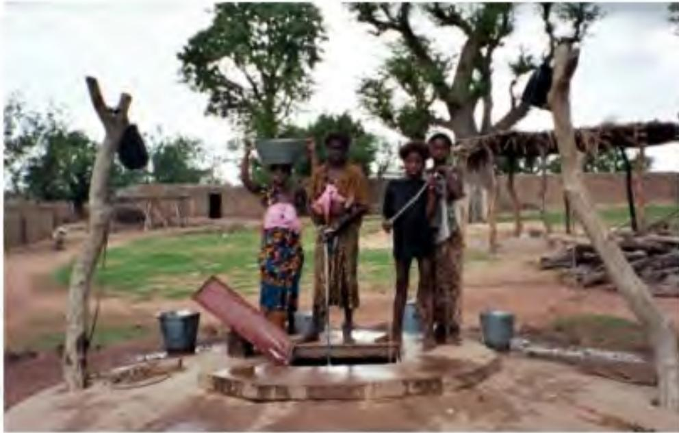
Figure 6: Girls pulling water from the completed well in Kodougouni. The reinforced slab with an access hatch and concrete apron are shown.
